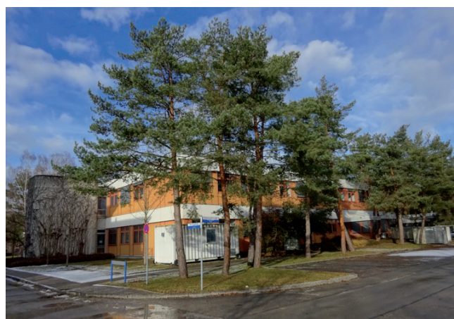
Figure 10: At the HMGU campus in Oberschleißheim (Building 24) JMSC/CMA operates climate chambers and special aerosol laboratories, partly in conjunction with the HICE MobiLab (see below).
